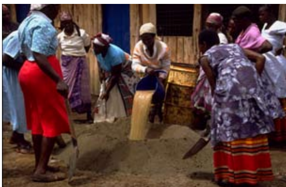
Harambee constructing water storage in Kenya
