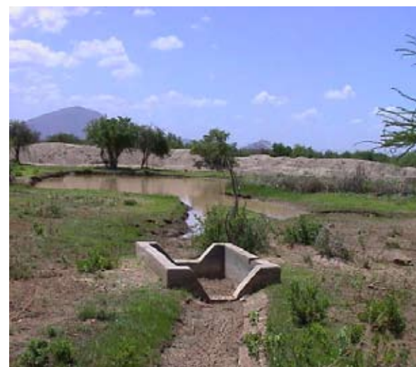
Photo (left): Silt trap intercepts sediments from the rainwater
