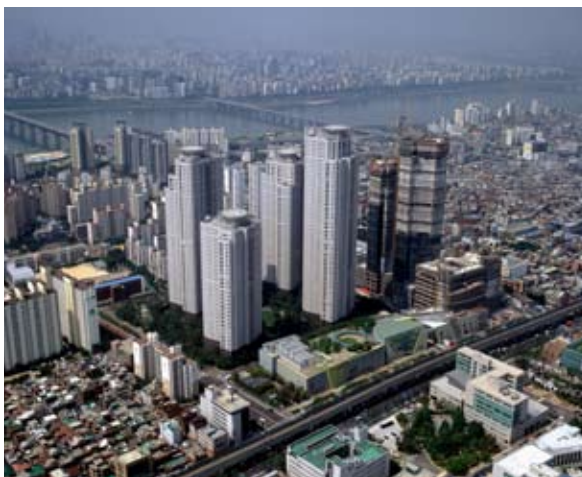
Site plan of the 4 towers, in total 6.25 ha in Seoul's City Centre, Korea POSCO
