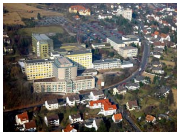
Aerial image of Bad Hersfeld Clinic, Germany. Harvesting rain from roof tops. Klinik Bad Hersfeld
