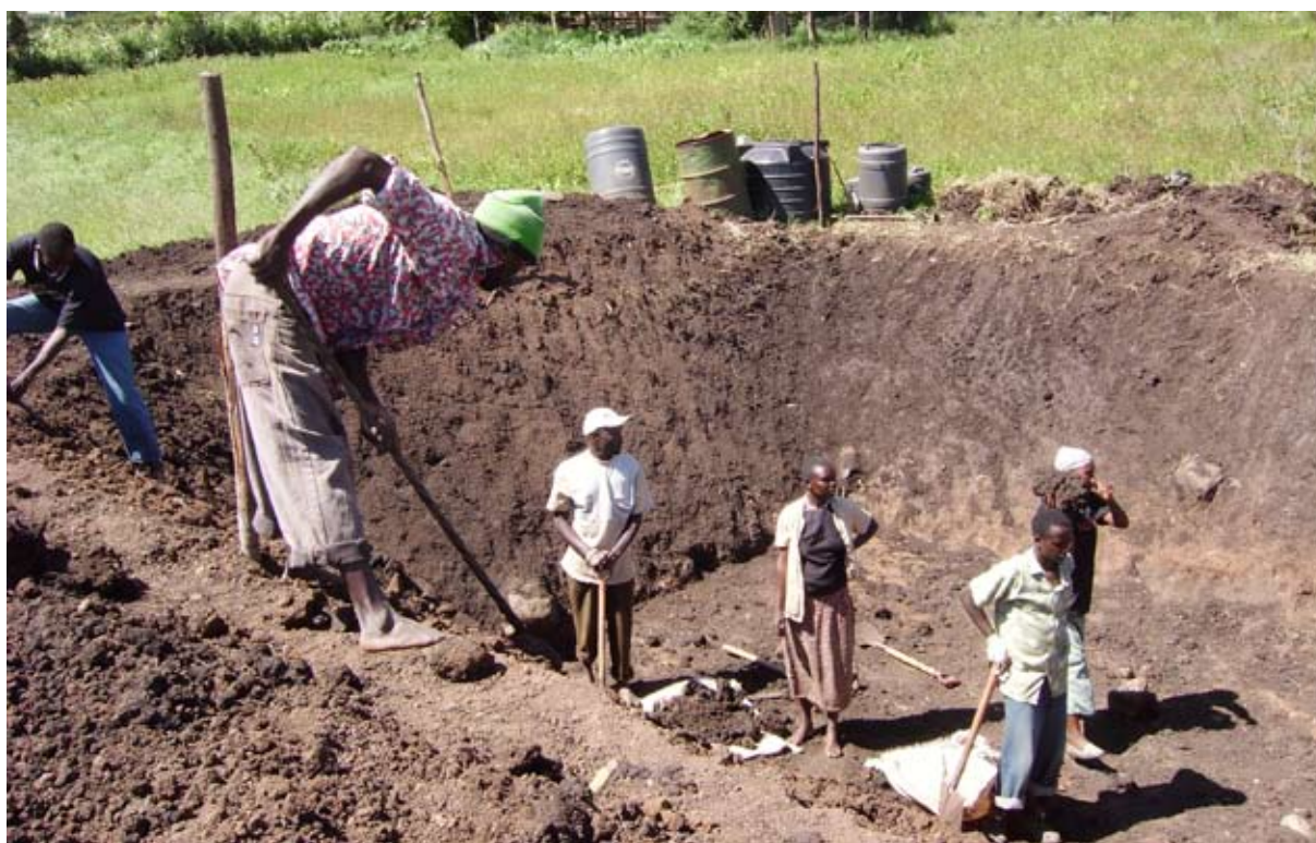
Working together to dig a runoff RWH pond
