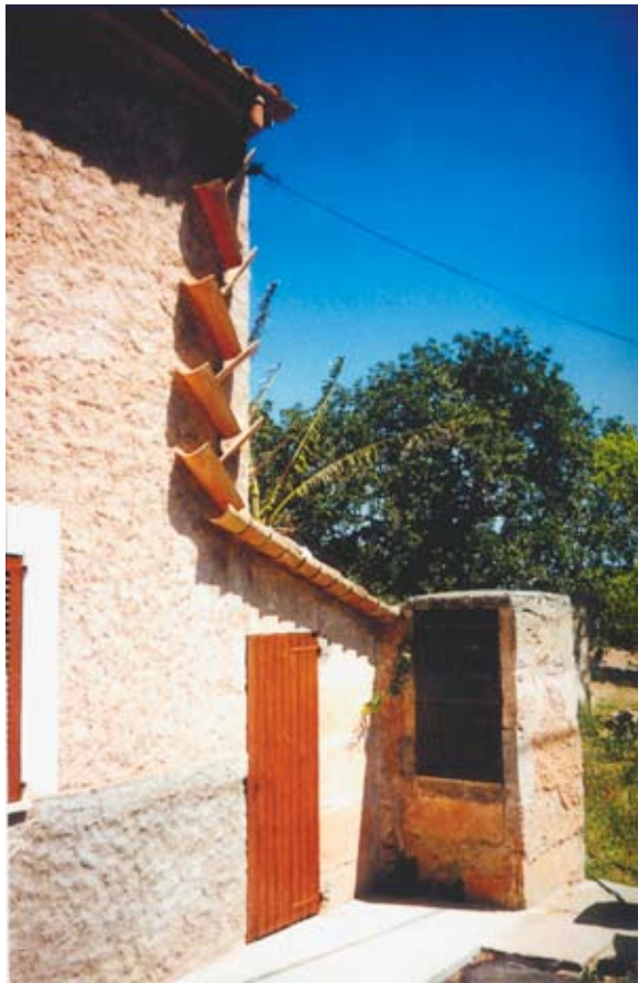
Rainwater Harvesting for domestic use on Mallorca Island, Spain
