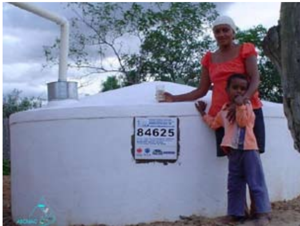
Tank no 84,625 in P1MC
